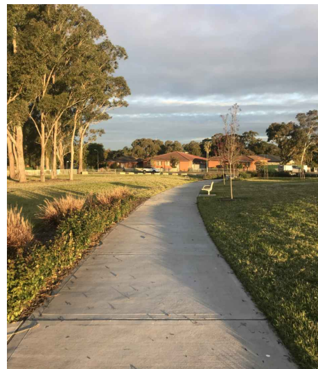
Concrete Footpath Broom Finished
